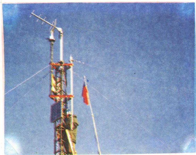
Photo 6. Installation of DCP in Punta Spring, January 1982.
