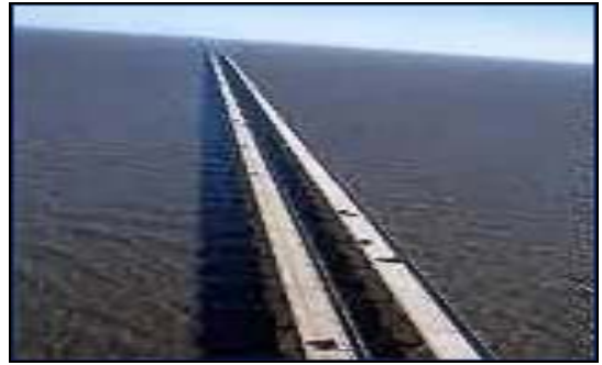
Fig.4 Aerial image of the Causeway bridge over the Pontchartrain lake.
